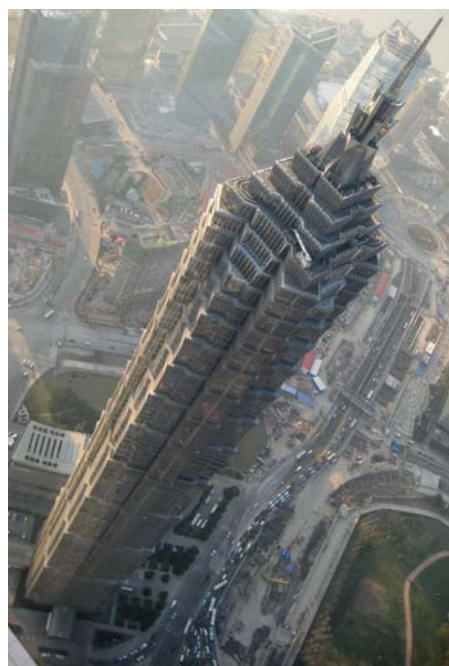
The Jin Mao Tower in Shanghai, China. Its exterior curtain wall is made of glass, stainless steel, aluminium and granite.
