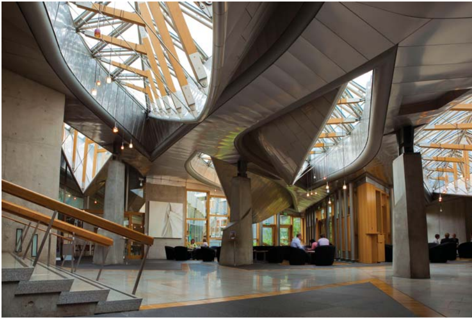
The garden foyer of the Scottish Parliament contains 12 skylights shaped like giant leaves. The roof glazing is supported by stainless steel connectors. Between the skylights are panels and coffers of stainless steel. Image © Scottish Parliamentary Corporate Body. Image © Scottish Parliamentary Corporate Body.
