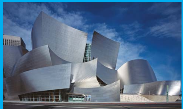
Designed by Frank Gehry, the Walt Disney Concert Hall, new home of the Los Angeles Philharmonic, is designed to be one of the most acoustically sophisticated concert halls in the world. Its stainless steel 316 skin is composed of convex and concave undulating surfaces.
