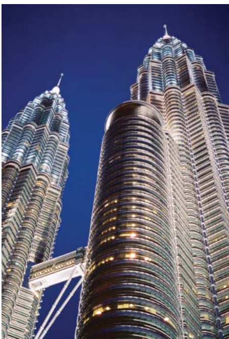
The Petronas Towers feature a diamond-faceted facade consisting of 83,500 square metres of stainless steel extrusions.
