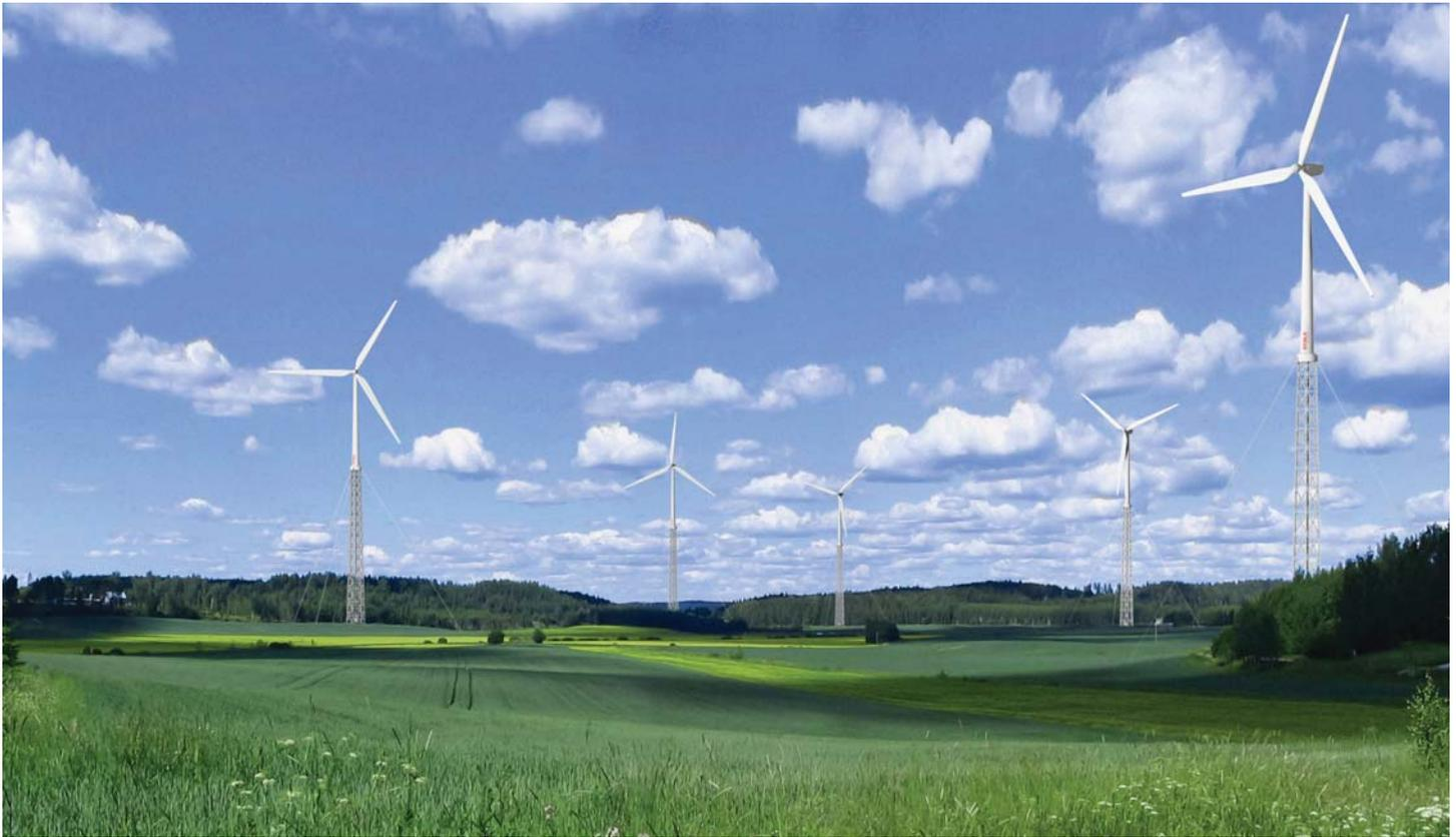
Stalutube selected Outokumpu's lean duplex grade LDX 2101® as one of the main construction materials for its new StalaWind wind power towers.
