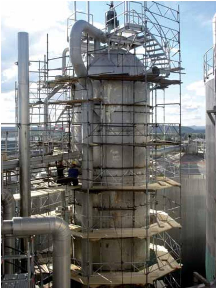
The hydrogen peroxide reactor under construction at Smurfit Kappa Kraftliner Piteå in Sweden at the end of August 2006 is the first industrial pressure vessel built out of LDX 2101®.
