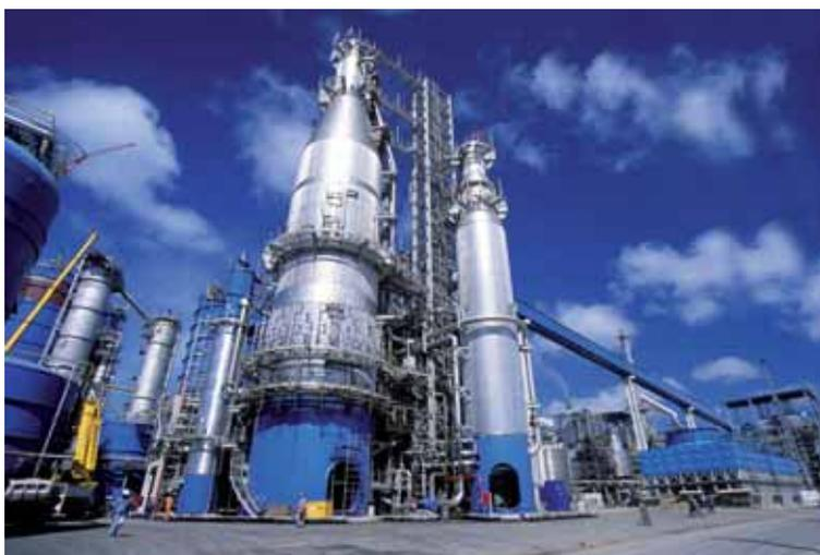
Metso Paper's continuous digester, installed in a plant in Brazil. Duplex materials are typically used in pulp mill fibre lines and particularly in pressurised vessels in cooking and oxygen delignification systems etc. Normally the material used in such digester systems is EN 1.4462, which is equivalent to North American S3 2205 standard. Source: Metso Paper.
